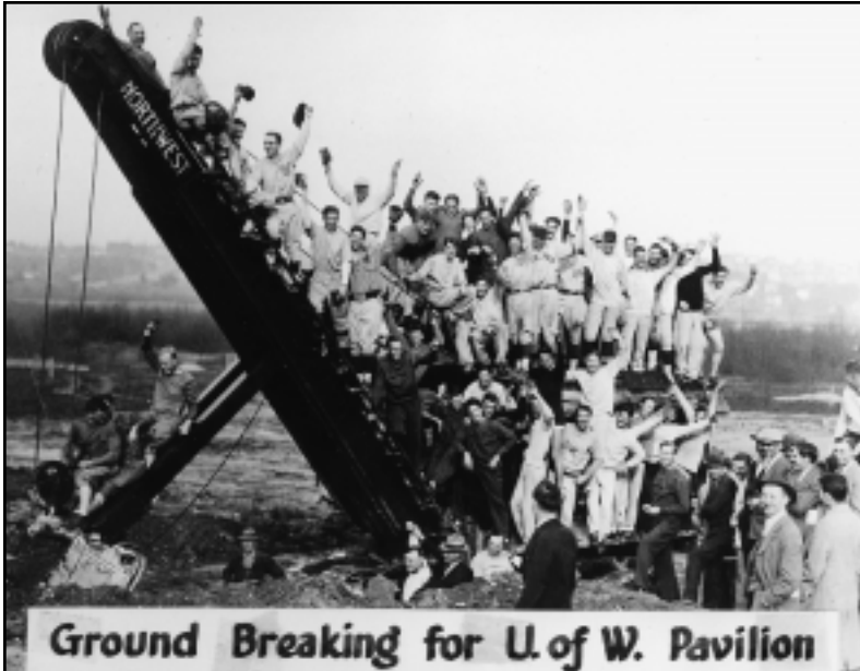
Husky athletes helped construction crews break ground for the Pavilion in early 1927.
